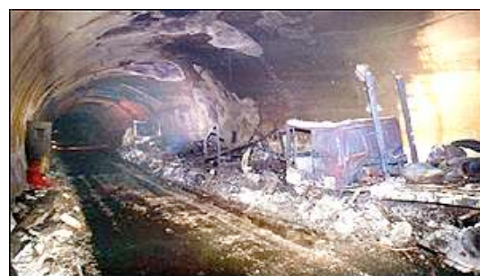
Aftermath of the Mont Blanc tunnel fire of March 1999 - the source of the fire was a truck carrying margarine and flour - the fire took 50 hours to completely extinguish
