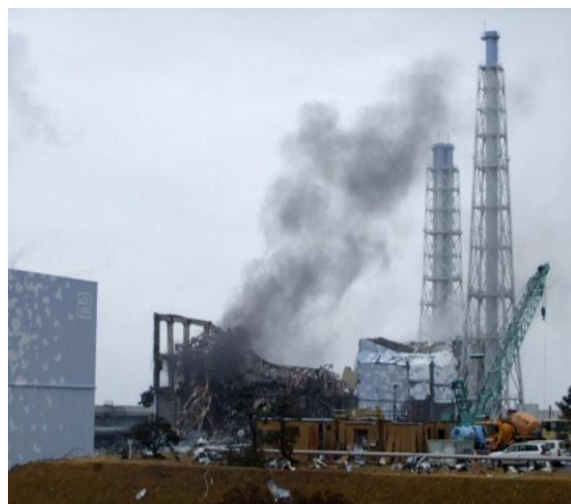
FIGURE 1 HULK OF THE CONTAINMENT OF UNIT 3 [centre]
