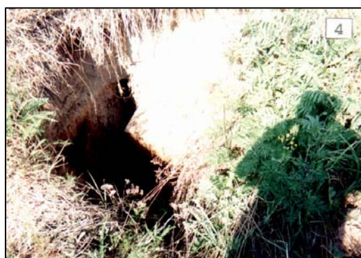
KOMPLEKSNY – VAULT AND PIT THROUGH CLAY CAP
