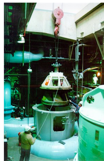
FIGURE 14 A MAIN CONDENSER COOLING PUMP , USUALLY ONE OF FOUR PUMPS
